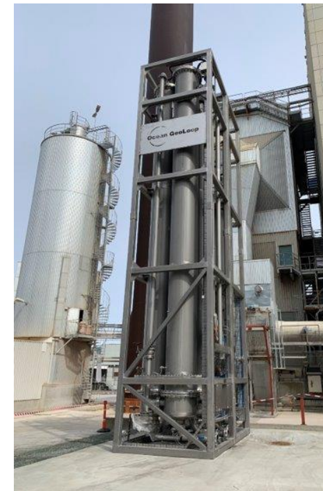
Pre-wash, absorber and desorber units installed at NSS April 2022
